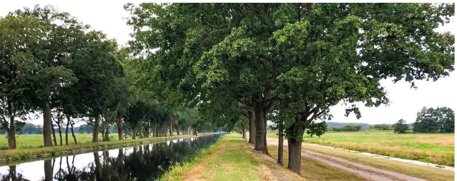
PHOTO The Stör-Canal is located in the middle of fields and meadows. Our ancestors were aware of the danger of dam fractures and developed a sophisticated flood protection system. This system of ditches, locks and weirs, completed in the 18th century, perfected in the 19th century and still maintained today, has worked well so far.
