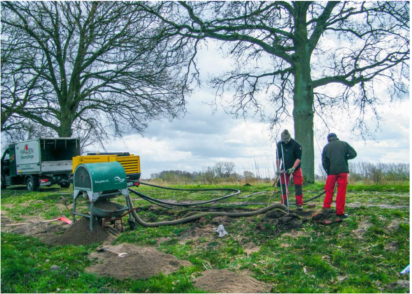
PHOTO Suction unit in use.
