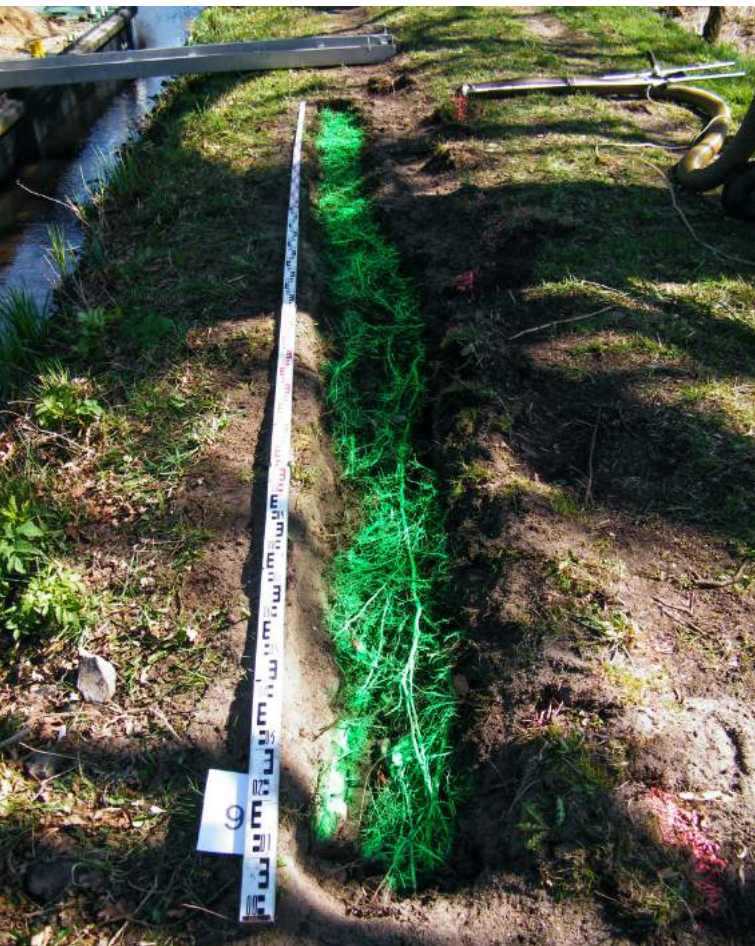
PHOTO Example root search excavation right bank Stör-Canal.
