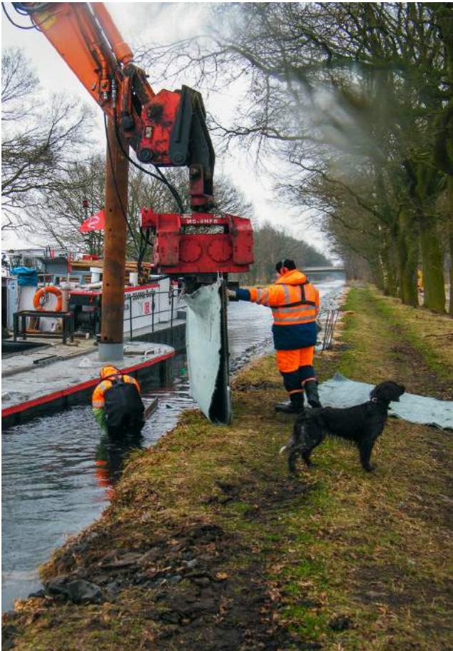
PHOTO Vibrating the fleece with a special device.
