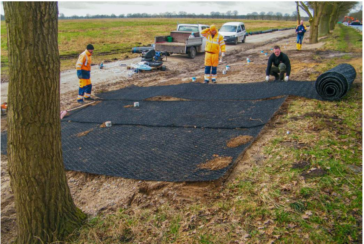
PHOTO Attaching the protective mesh against burrowing animals.
