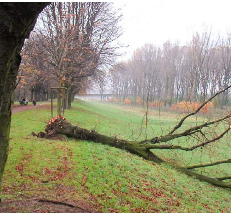
PHOTO Stability failure in the storm due to missing tree control.
